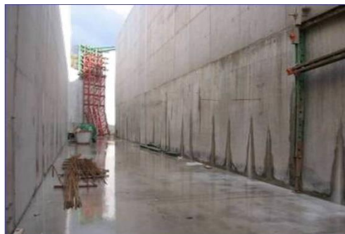
Figure 3. Thermal shrinkage of reinforced concrete walls (Al-Gburi, 2014) .
