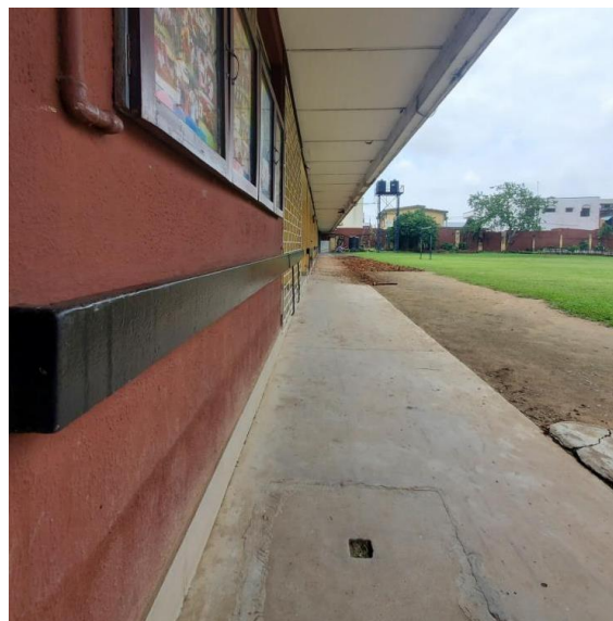
Figure 7. Handrails to support students in the school corridor.
