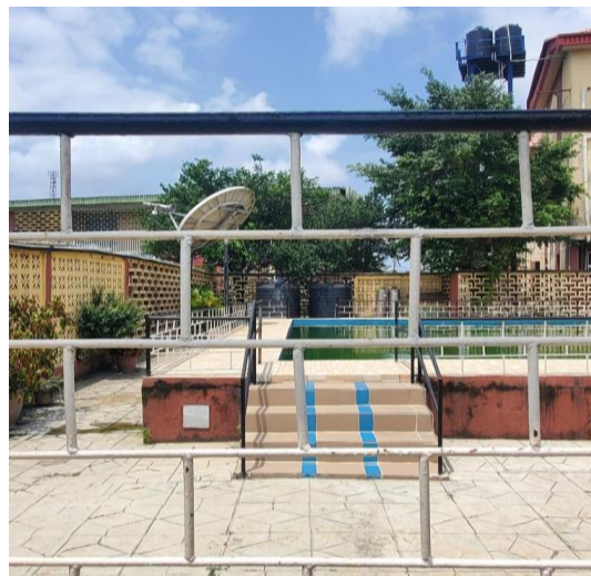
Figure 5. School Swimming Pool.
