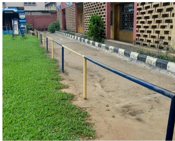
Figure 3. Recently added handbars to support students near the playground
