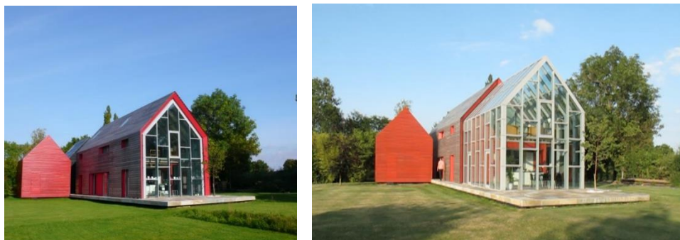
Figure 2 Sliding house with horizontal transformation
