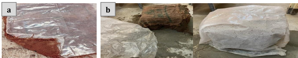
Figure 10. Damp-burlap (DBC): (a) Burlap coated with polyethylene sheet, (b) Immediately after casing
